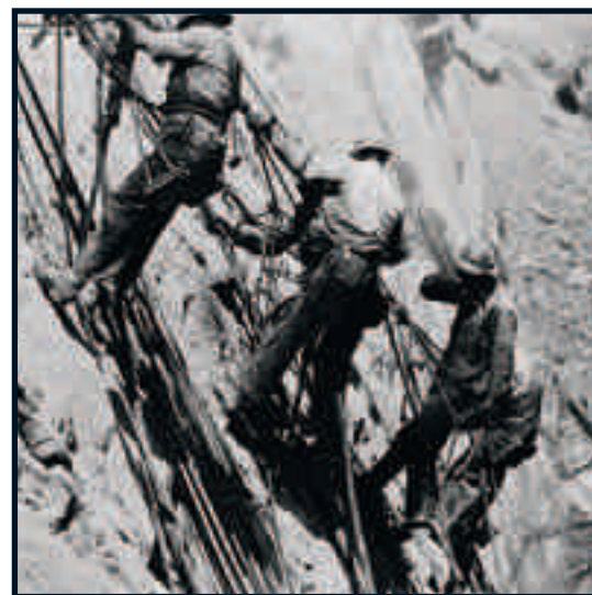
Suspended on ropes, “high scalers” armed with dynamite and jackhammers prepare the walls of Black Canyon to take the concrete of Hoover Dam. Such work was hazardous. Twenty-four workers fell to their deaths during construction of the dam.
