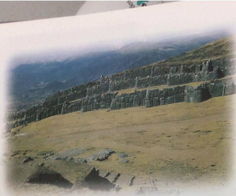
The 50-foot-tall stone walls of Cuzco were built without mortar by the Inca.
